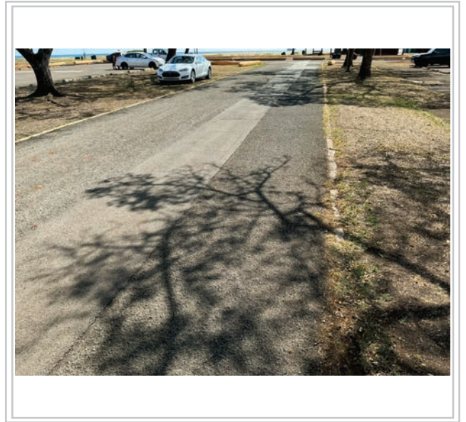
Area to be repaved
