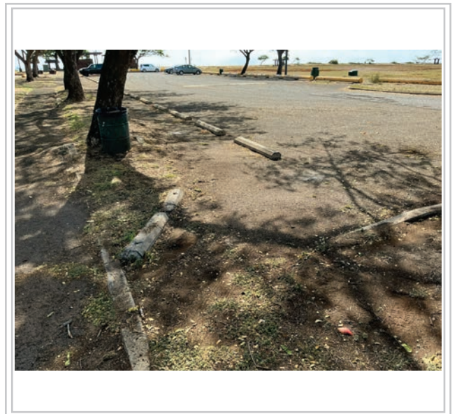
Area to be repaved
