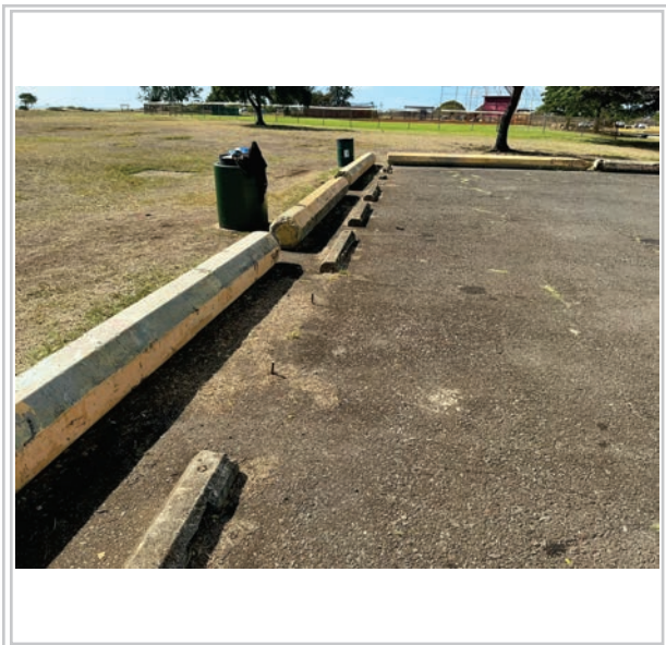
Area to be repaved
