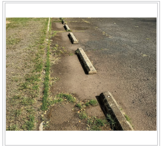
Area to be repaved
