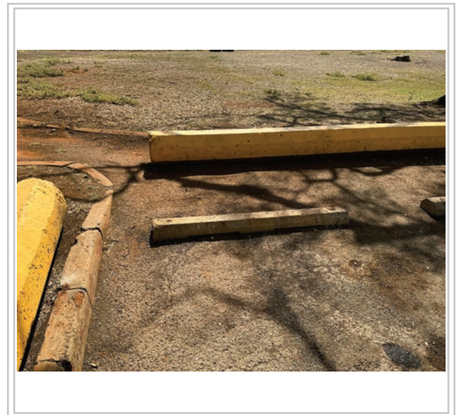
Area to be repaved
