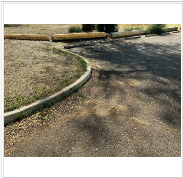
Area to be repaved
