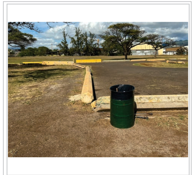
Area to be repaved
