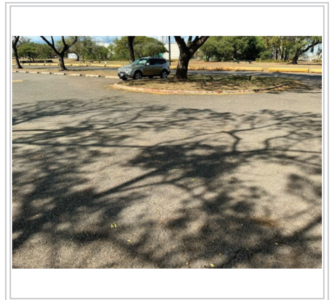
Area to be repaved
