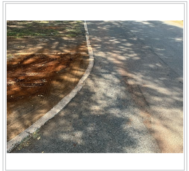
Area to be repaved
