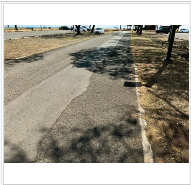
Area to be repaved
