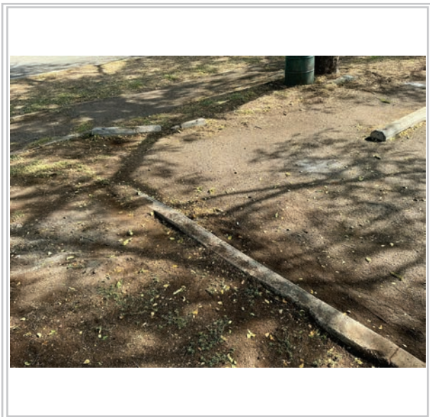
Area to be repaved
