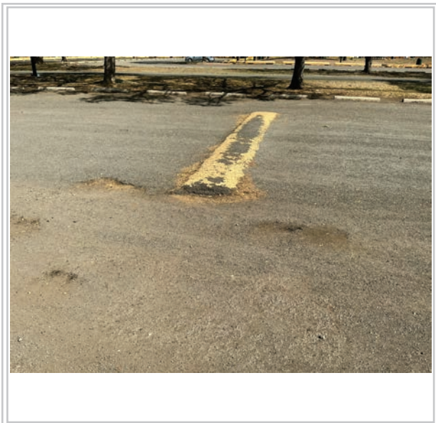
Area to be repaved
