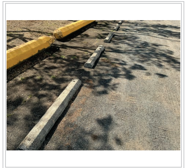
Area to be repaved
