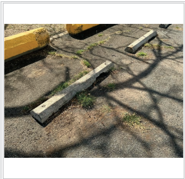
Area to be repaved
