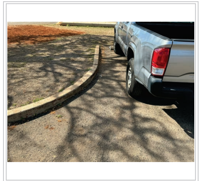
Area to be repaved
