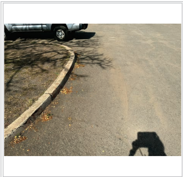
Area to be repaved
