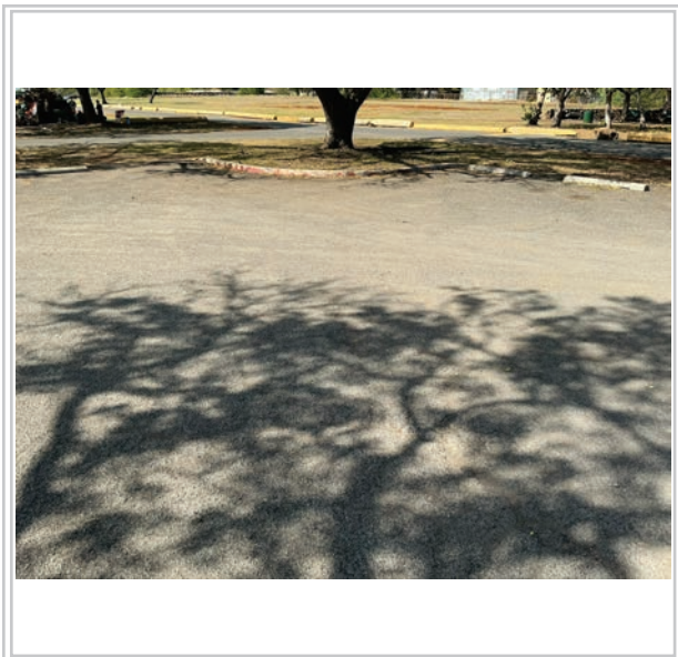
Area to be repaved
