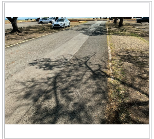
Area to be repaved
