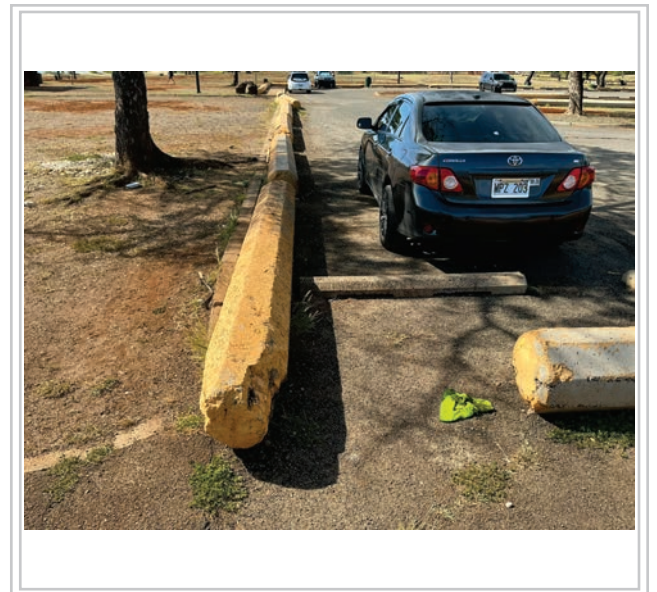
Area to be repaved
