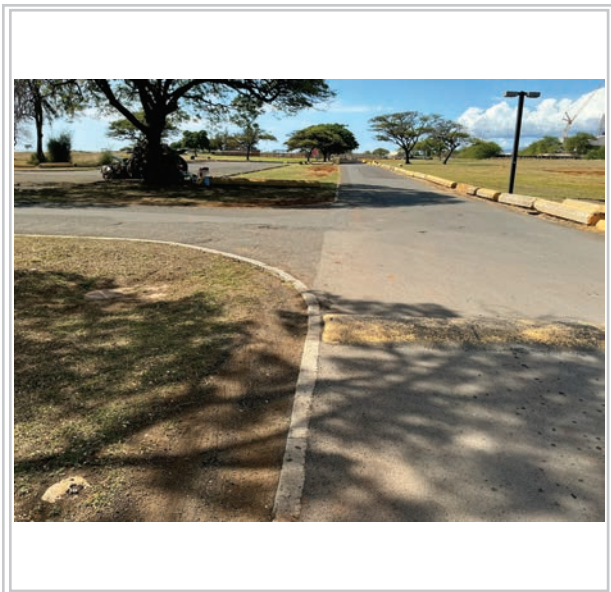
Area to be repaved
