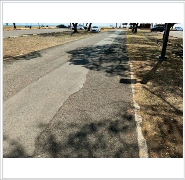
Area to be repaved
