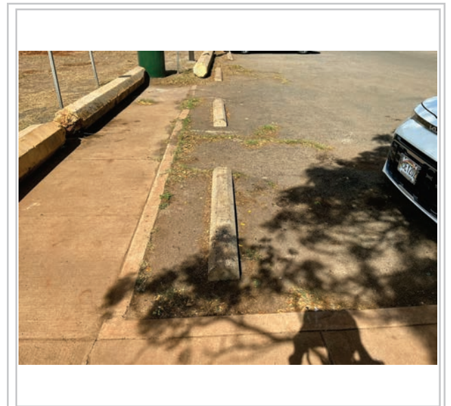
Area to be repaved
